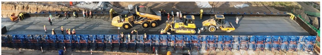
Figure 5. Construction of the FSTE
